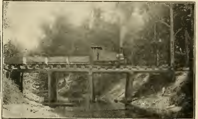
RAILWAY BRIDGE IN NORTH BORNEO, WITH BALLAST TRAIN CROSSING.
